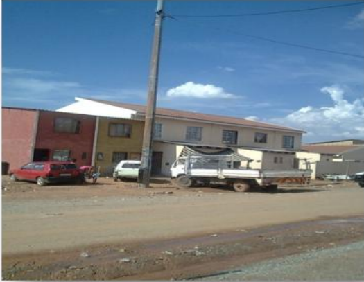
Photo 2: In Sol Plaatjies former mine housing units were being converted into duplex semi detached houses (Photo taken by author)
